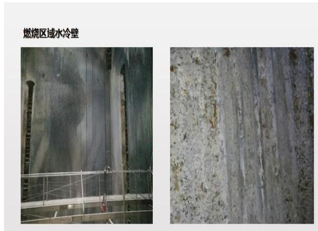
图5水冷壁管形貌
